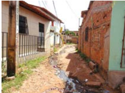
Beco com esgoto a céu aberto Alley without sewage system
